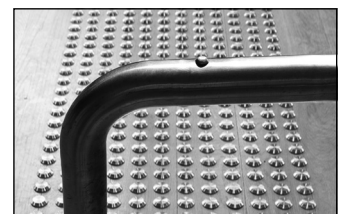
HANDRAIL TACTILE INDICATORS
